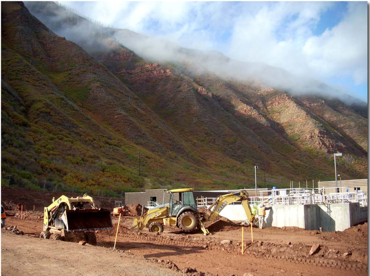
SITE GRADING TO FINAL ELEVATIONS
