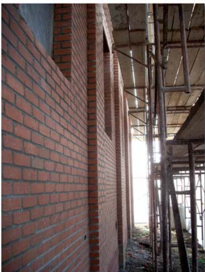
LIFT STATION BRICK VENEER
