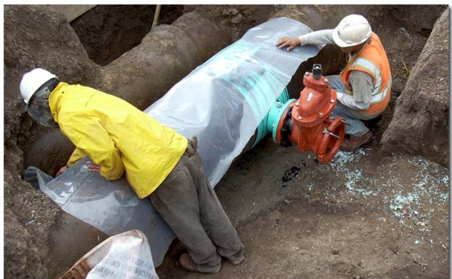
COMPLETING 8-INCH TAP OF 24-INCH RAW WATER LINE
