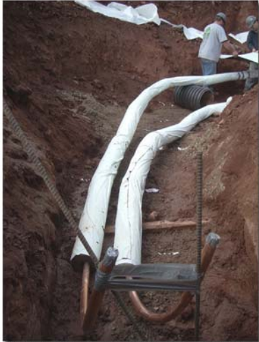
INSULATING GROUND SOURCE HEAT PIPING
