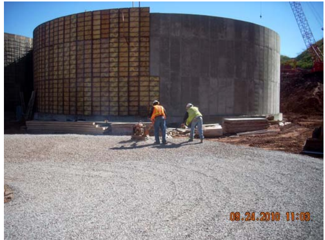
Preparation for Clarifier Slab - South O-Ditch Behind
