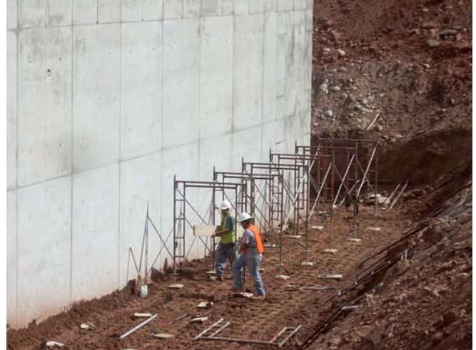
Erecting Scaffold - Digesters Masonry
