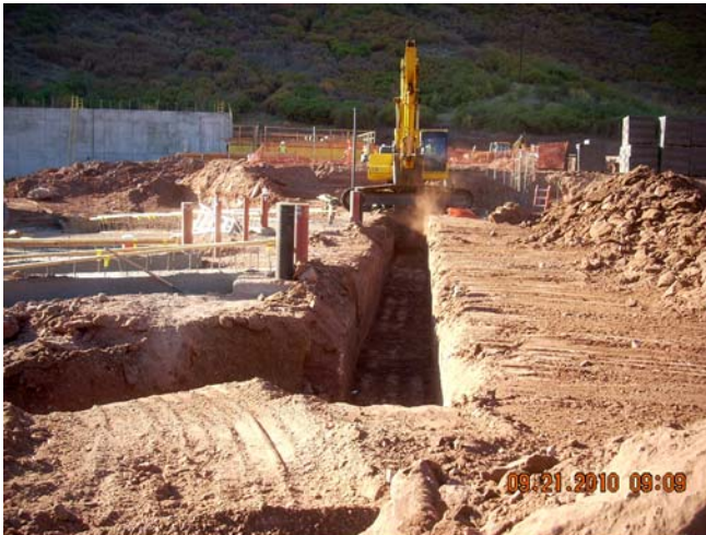
Underslab Piping at RAS Building
