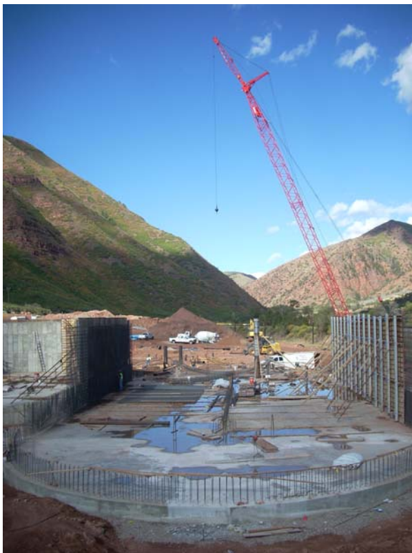
Concrete Placements - Digester Tanks to Left; Oxidation Ditches to Right
