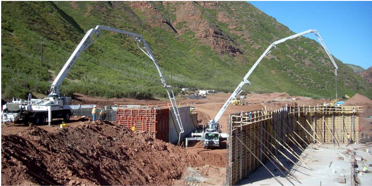
Concrete Placements - Digester Tanks to Left; Oxidation Ditches to Right
