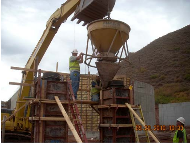
Clarifier Influent Pipe Encasement
