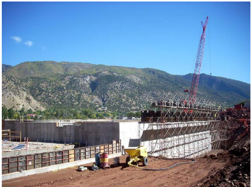
Masonry work began September 22
