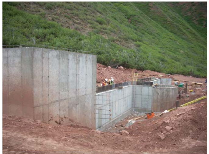
Headworks Building - August 16
