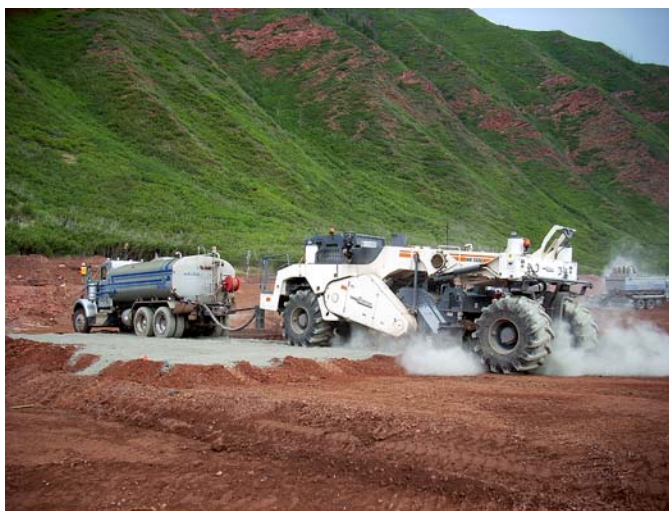
Blending cement with Soil - Maintenance Building
