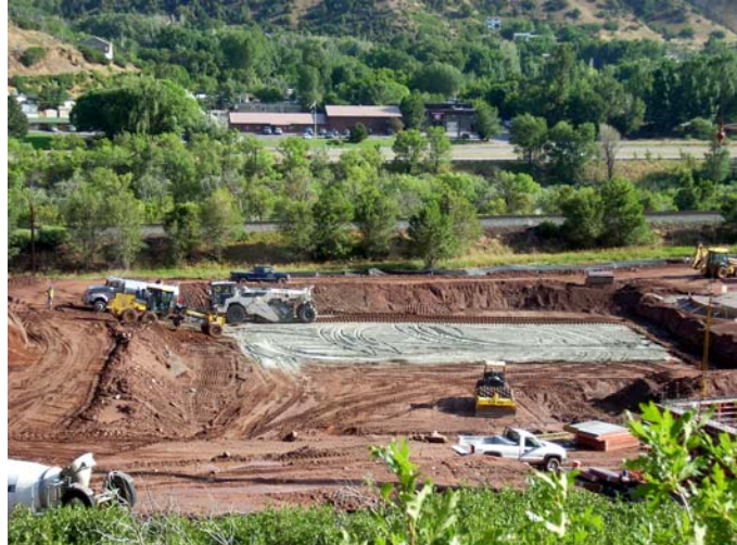
Cement treated soils operations at the Clarifiers Structure
