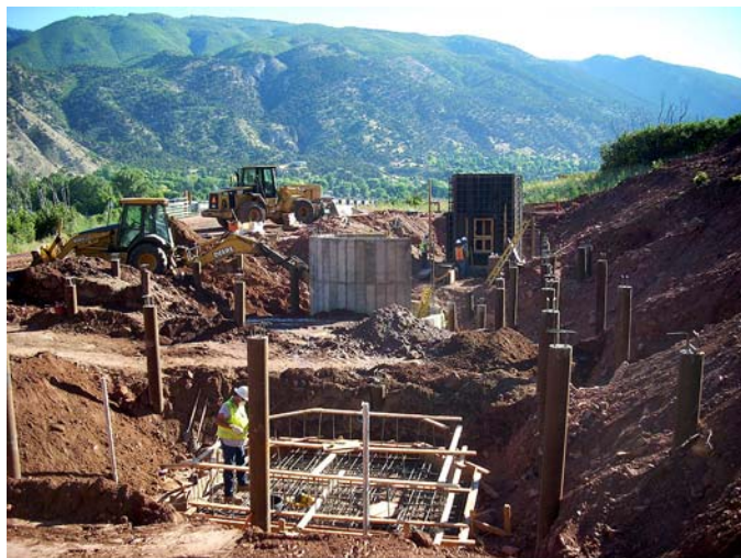
Headworks - Pipe piles completed some 50+ feet Deep
