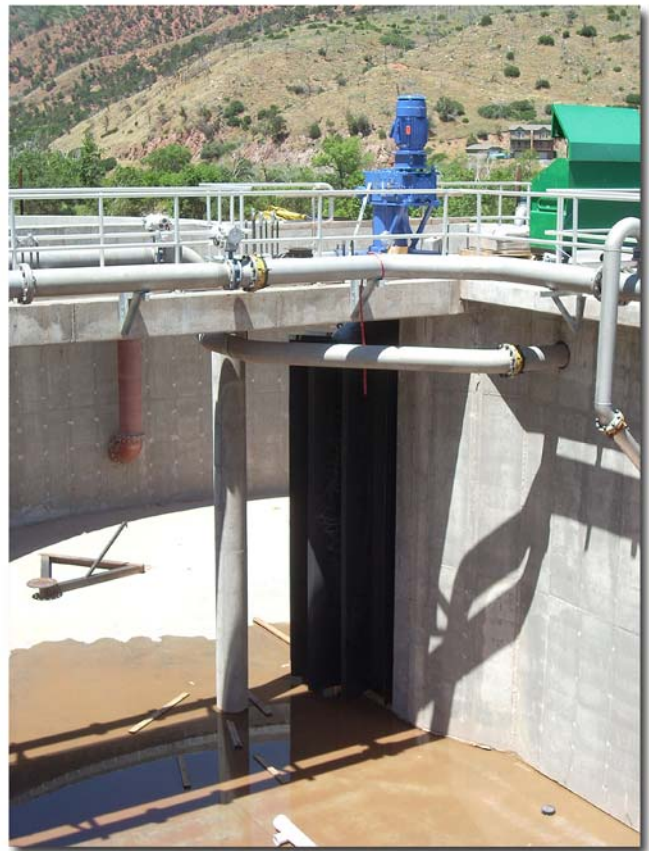
Oxidation Ditch - Vertical Drum Mixer
