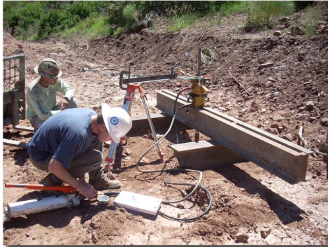
Micropile Verification Testing - Rockfall Fence
