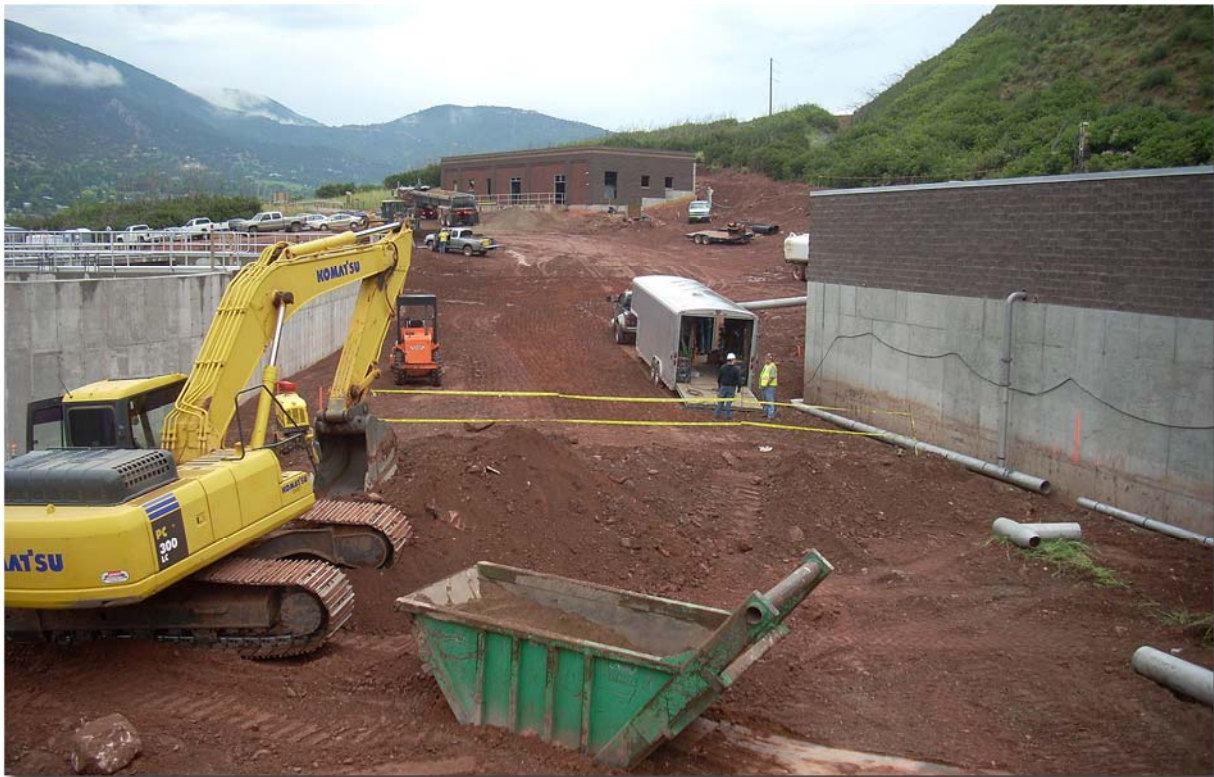
Installing Stainless Steel Pipe North of Digesters
