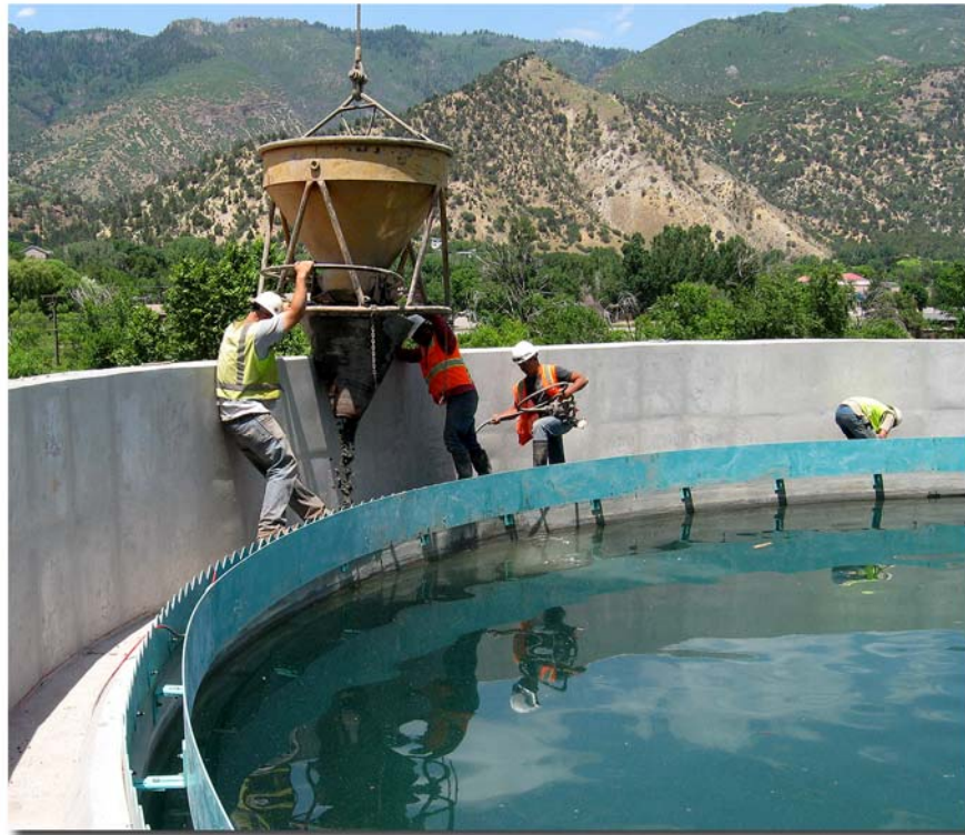
Placing Grout Invert in Clarifier Effluent Trough
