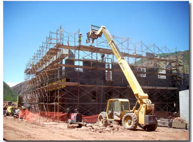
Administration Building - Masonry
