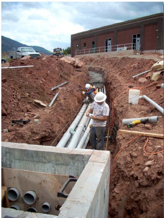
Main Electrical Feed to Plant - Ductbank Installation
