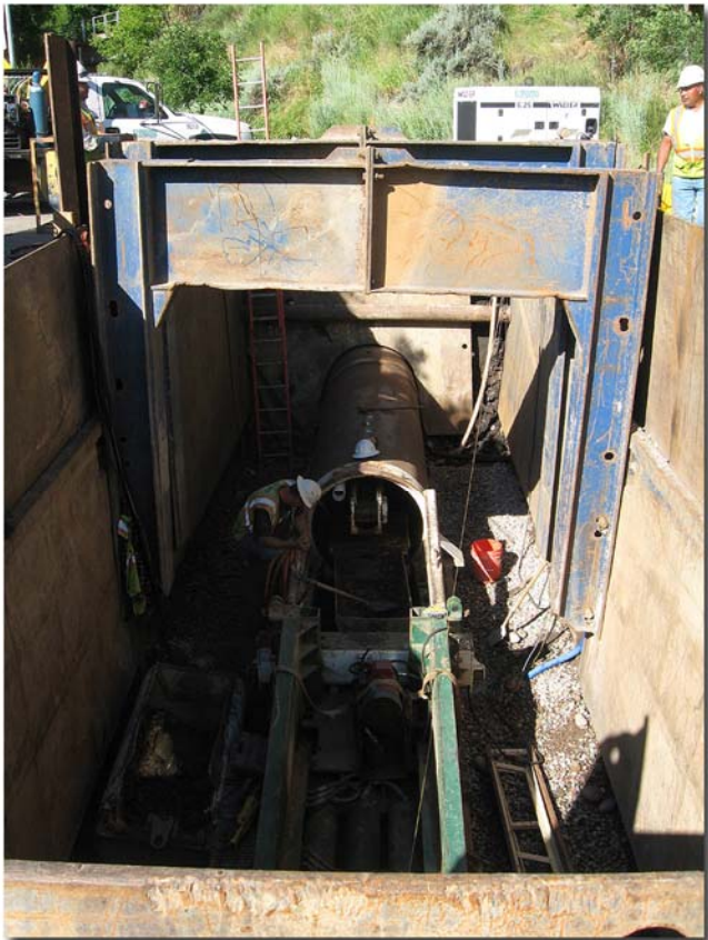
Installing Casing thru Bore Under RFTA Tracks
