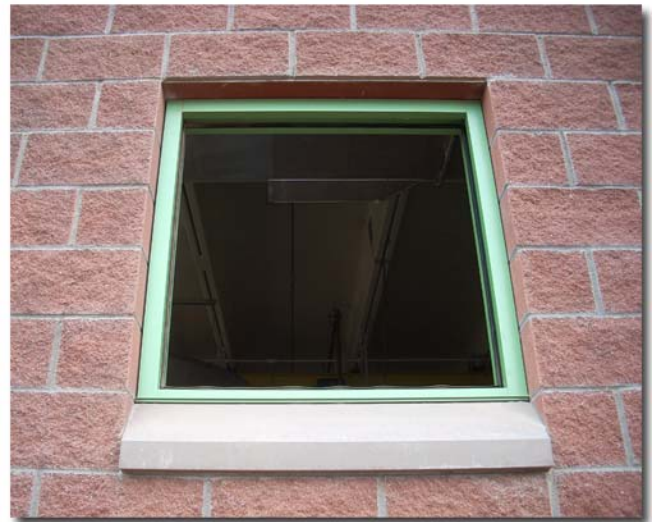
Window Frame Installed
