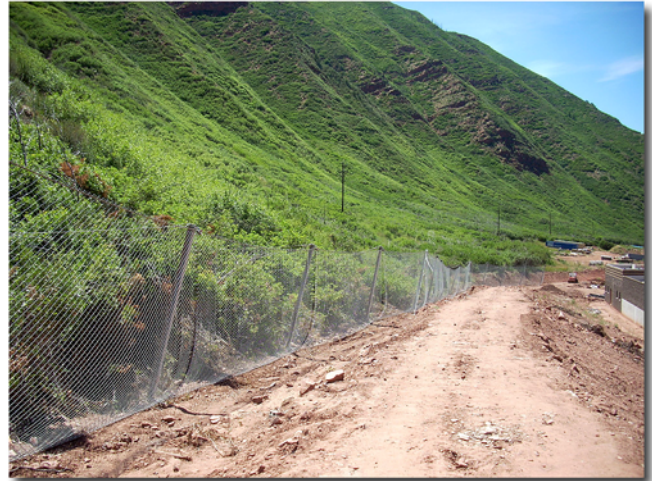
Rockfall Protection Fence at South Side of Facilities
