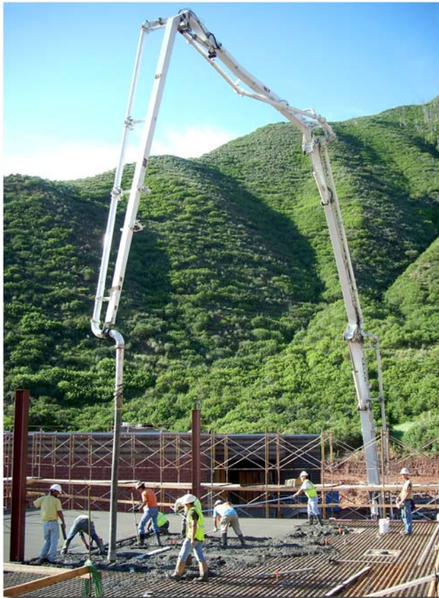
Admin Building Upper Level Deck
