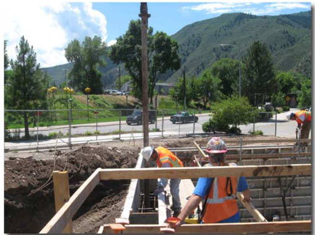
Lift Station - Concrete Wall Placement
